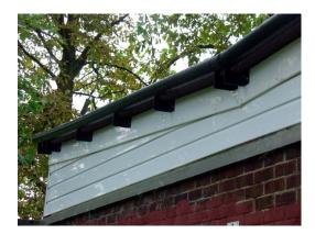
The standard system consists of a single row of rotating cups threaded onto a central shaft.
