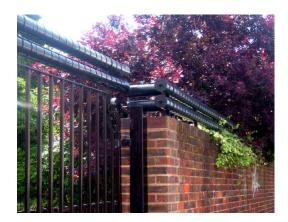
There are however occasions, such as where Roller Barrier is needed as an anti-climb barrier for mounting on a low wall or fence, where a single row of cups may not prove an adequate deterrent.
