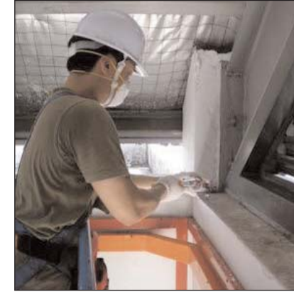
position dishes at edge of beam or sill
