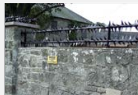
Perimeter Walls & Gates
