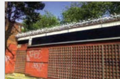
Community centre roof
