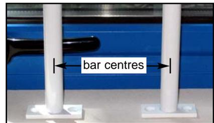
Now, using a tape measure, measure from the centre of your window out to the right ...at every 100mm point you'll need a bar (if it's a Child Safety Application), or at every 150mm for a security application. (Remember: the distance between the edge of the window and the centre of the bar closest to it should'nt be any greater than your chosen bar centres).
