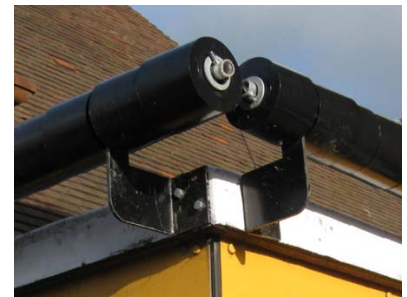
outward facing corner installation
