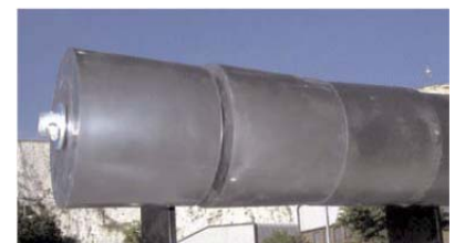
At the end of the installation, the last cup should be installed to show a solid outward facing face.
