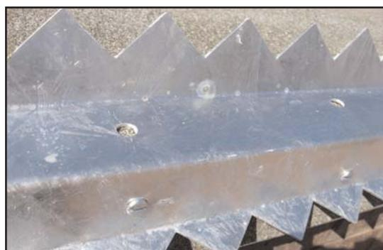
...face fixed - installed around the edge of a flat roof
